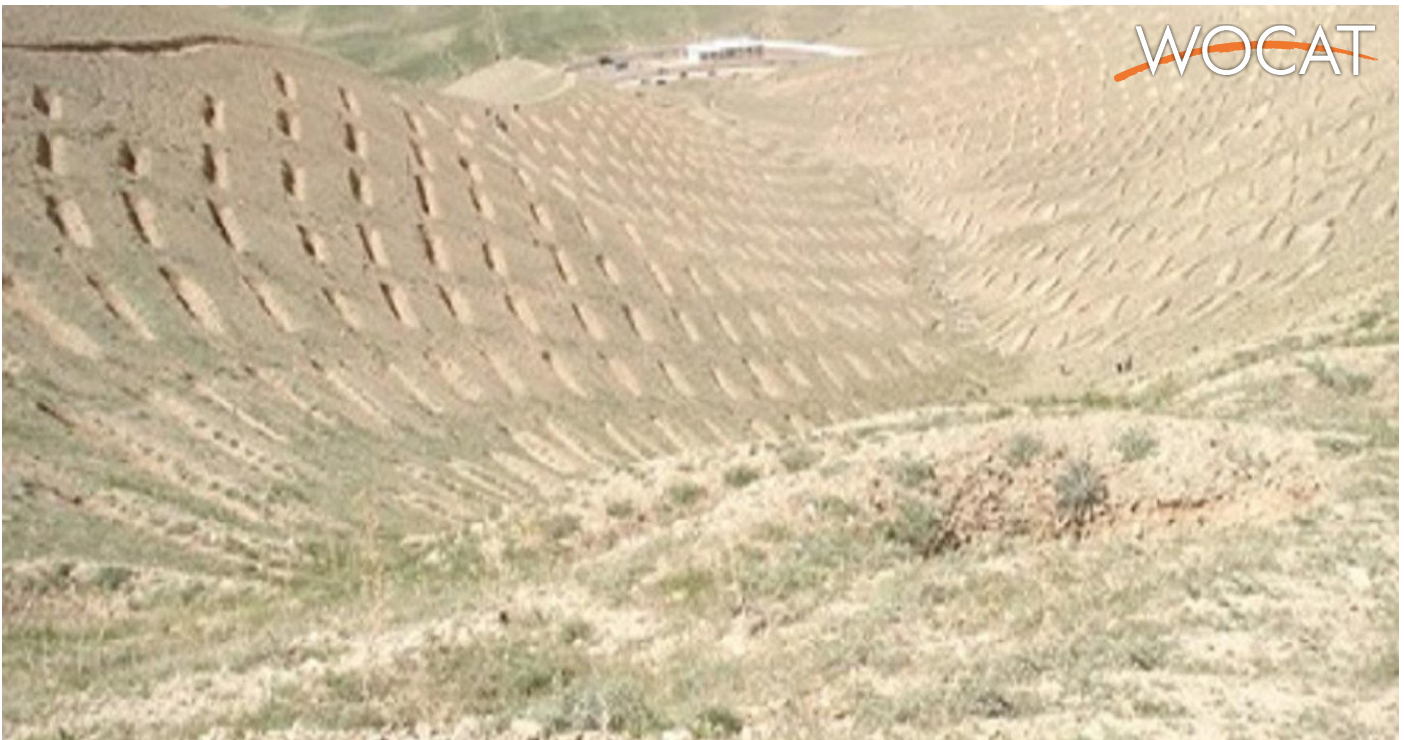
An overview of the staggered contour trenches applied across the slope on a hilly slope of Zai Mahmood village in Bamyan center. (Jalil Altaf (Agha Khan Foundation (AKF)))
